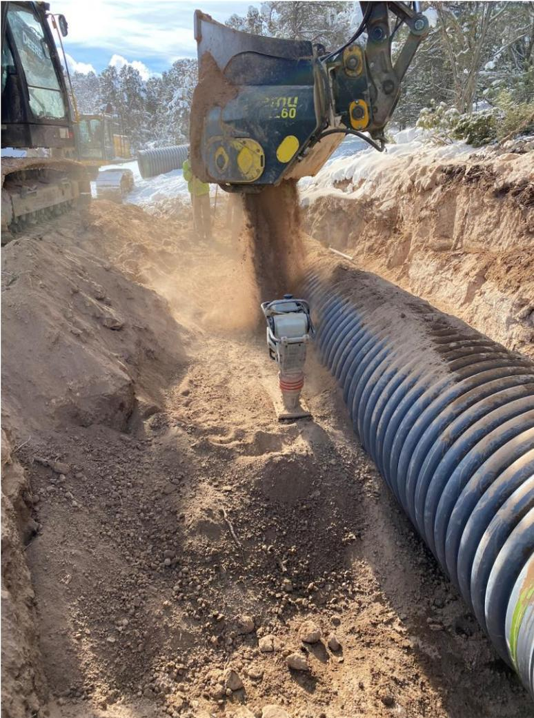
*Figure 12. Backfilling Pipeline on Section Two of the Gould Canal Improvement Project B - in Crawford, Colorado*
