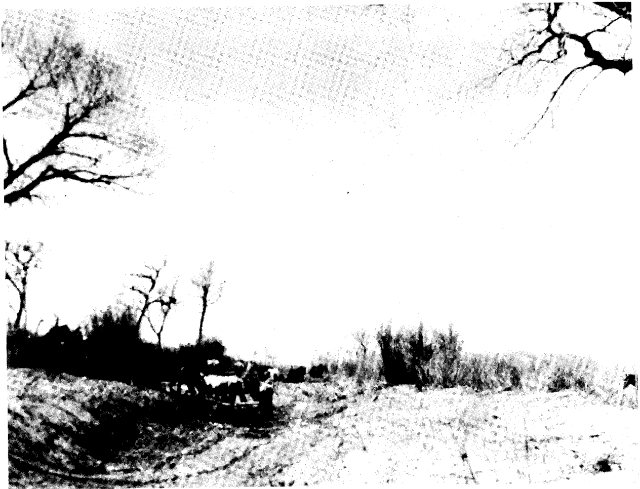
Horse drawn go-devils and scrapers were used to excavate canals. (Photograph courtesy of Fort Duchesne, 1922.)
