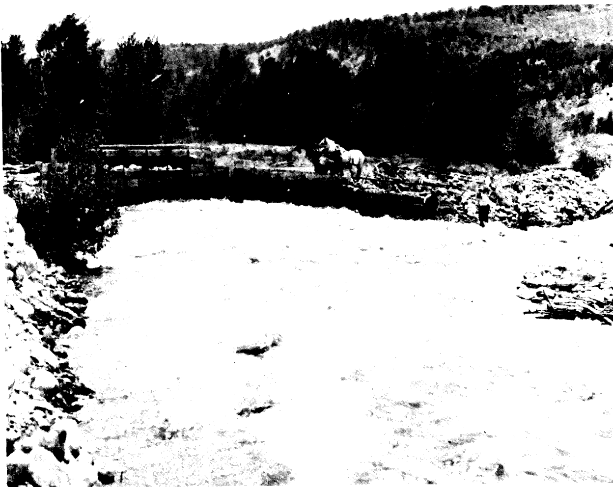
Unusually high water in June of 1930 threatened the headgates of the Lake Fork Canal. Here employees of the Dry Gulch Irrigation Company with teams of horses are attempting to remove debris from the inlet channel. (Photograph courtesy of Fort Duchesne, 1930.)
