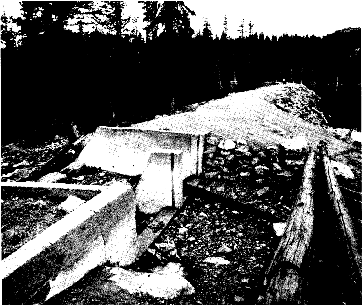
Concrete spillway with freeboards removed and remnants of log trash rack on Wall Lake Dam. The dam was built by the Provo Reservoir Company using crews of farmers from the Heber Valley.
