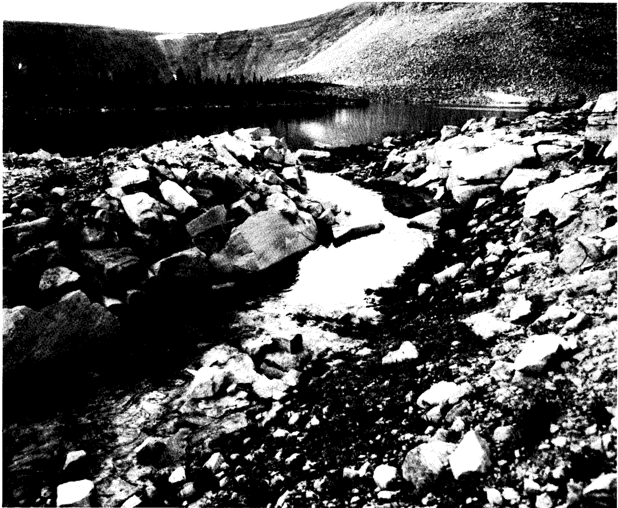
Rock-lined spillway of Drift Lake Dam, a high mountain lake in the Yellowstone River drainage.
