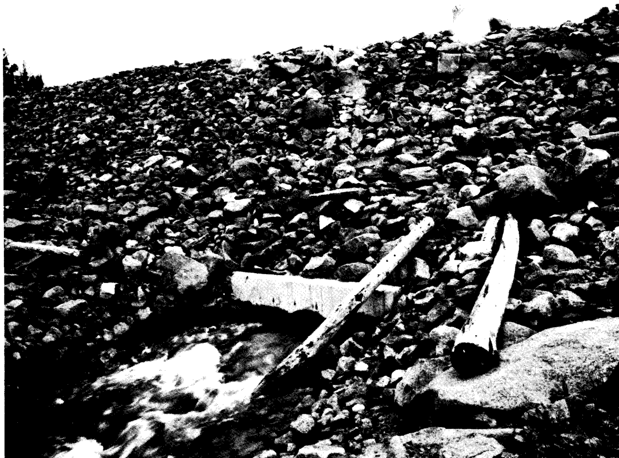
Downstream outlet gate and collar on Clements Lake Dam, the largest and highest of the four Lake Fork River reservoirs. It is the only reservoir constructed by the Dry Gulch Irrigation Company in the Lake Fork drainage.
