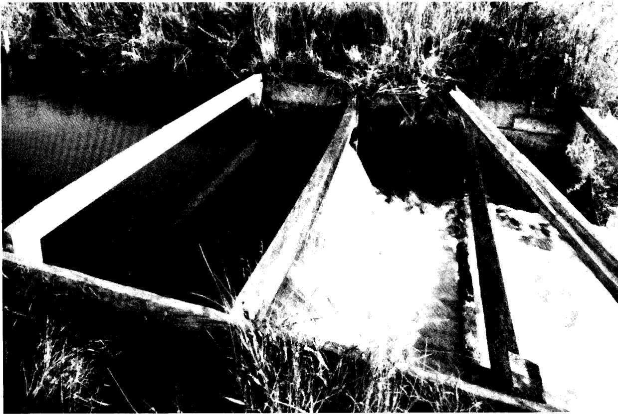
Measuring weirs such as this box on the U.S. Deep Creek Canal helped to ensure that each landowner received his fair water allotment.
