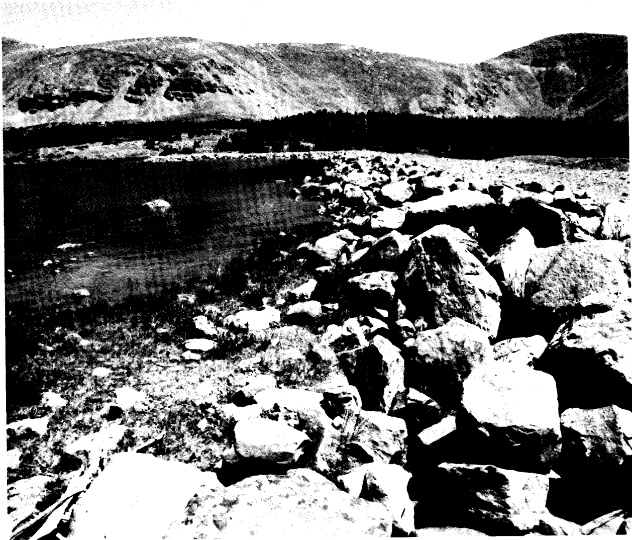
Upstream face of East Timothy Lake Dam, the largest dam in the Upalco Unit and the last privately financed dam in the Swift Creek drainage. The original rudimentary sod dam constructed by Brigham Timothy c. 1920 was replaced by the Moon Lake Water Users Association in 1951 by the present extensive earth-fill structure.
