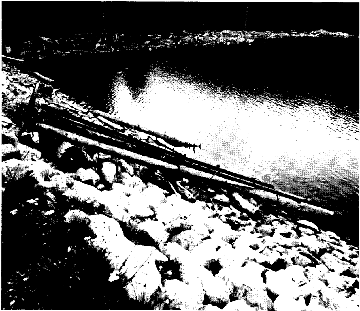
Inclined outlet gate, wheel, stem, and stem guide at Duck Lake Dam.
