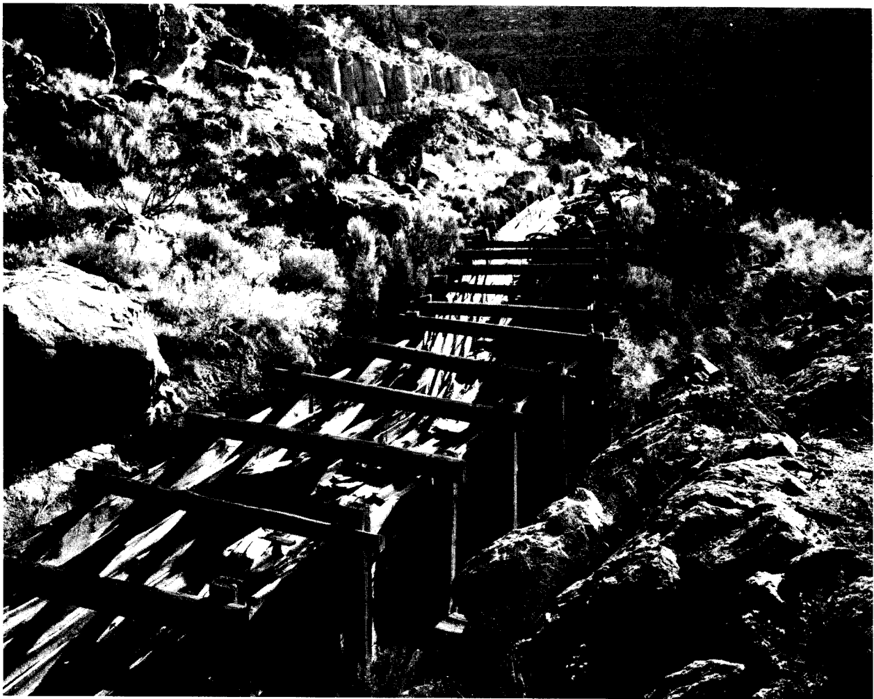
The serpentine Knight Ditch flume guided water over rugged sage brush covered terrain to irrigate farlands on the Blue Bench.
