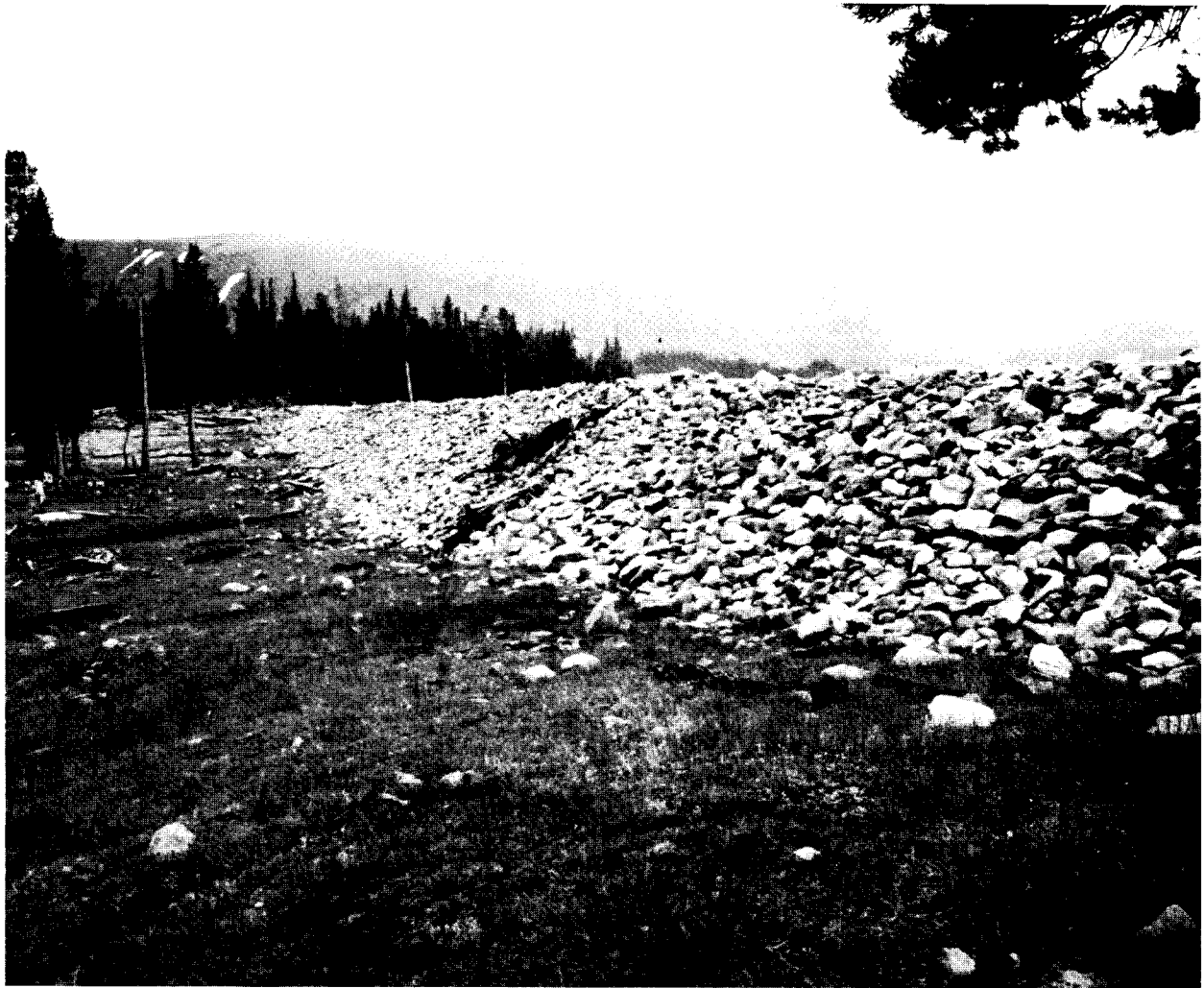
Downstream face and toe of Kidney Lake Dam. The largest of the impounded high mountain lakes in the Upalco Unit, the reservoir was one of three lakes in the Brown Duck Basin dammed by the Farnsworth Canal and Reservoir Company.
