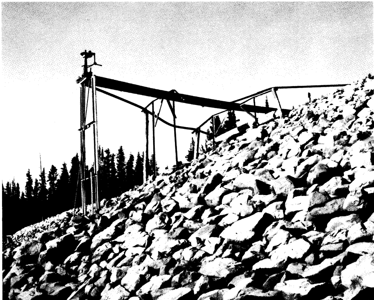
Upright outlet gate, wheel, stem, and stem guide at Lost Lake Dam.
