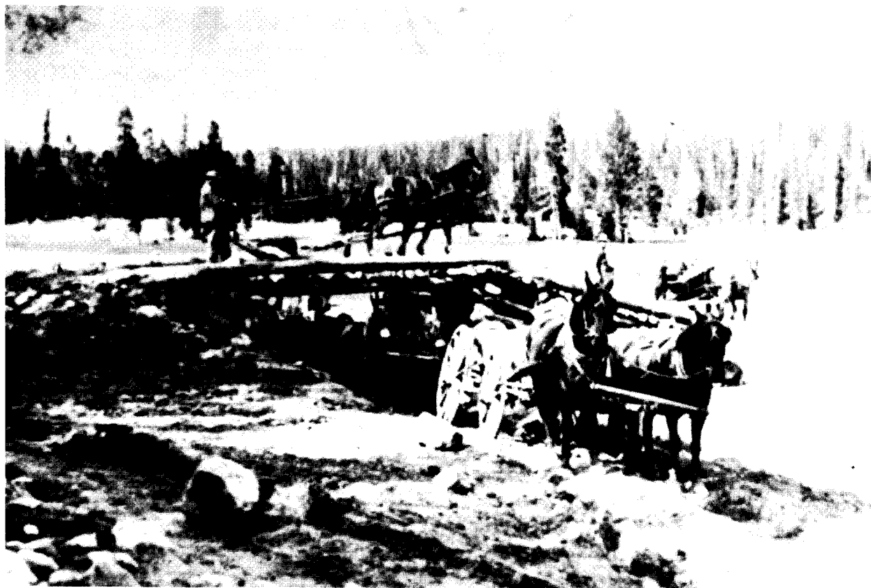
Construction at Lost Lake Dam showing loading platform. Lost Lake dam is the largest of the earth-fill retention structures. Construction required more than 60 men, 8 teams, and several large trucks. (Photograph courtesy of Ardean Anderson, Kamas, Utah, September 7, 1912.)
