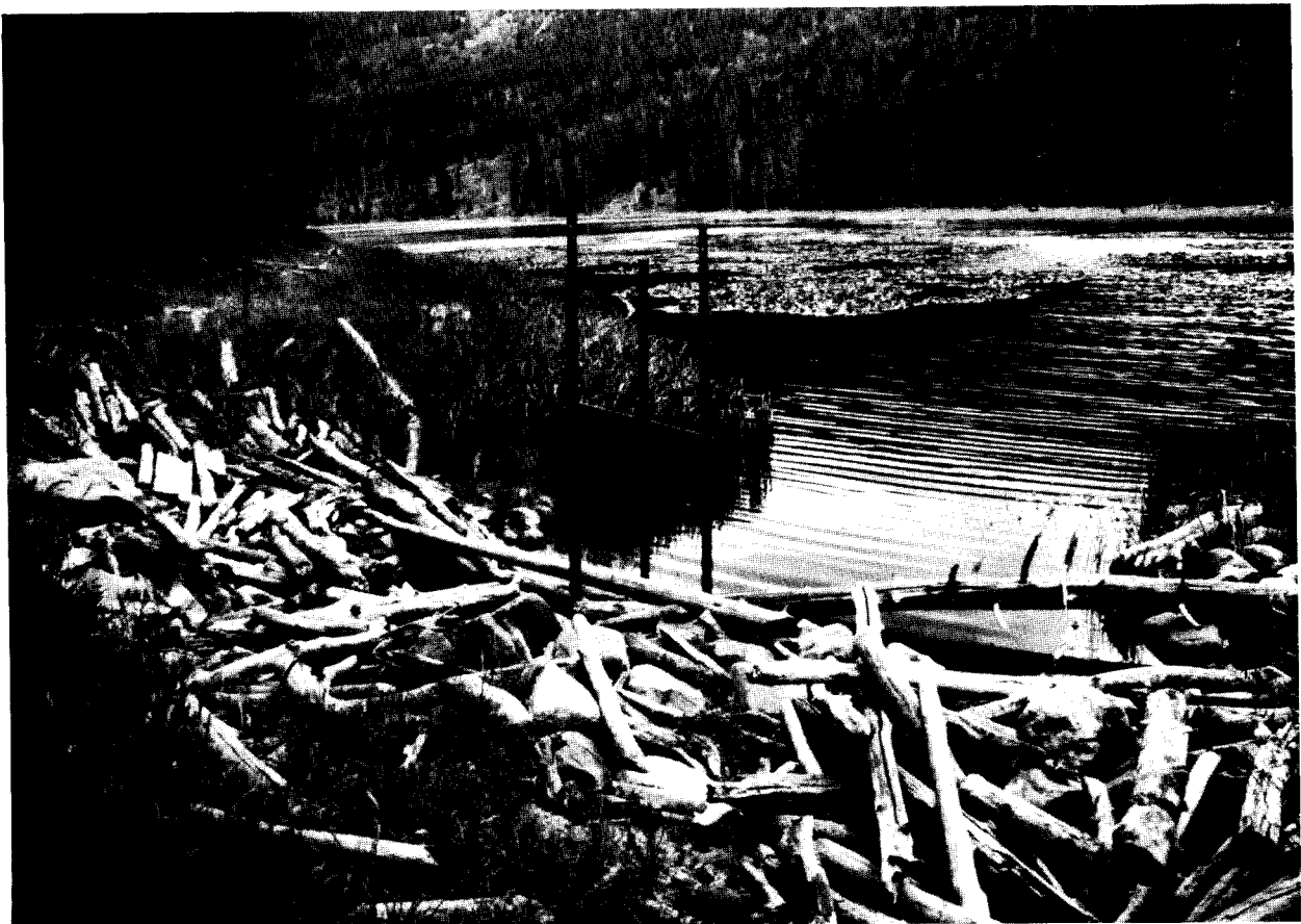
Upstream face of Water Lily Lake Dam shows upright (inoperable) outlet gate. Water Lily is the smallest of the dams in the Upalco Unit as well as the oldest man-made structure to reservoir a natural lake in the Swift Creek drainage.
