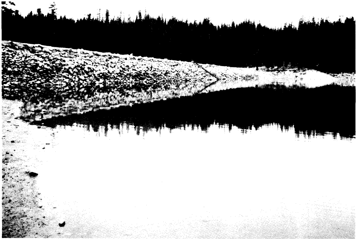
Upstream face of Trial Lake Dam. The dam, was technologically notable for having a concrete core. The present 1914 dam followed an 1899 failed attempt to dam Trial Lake.
