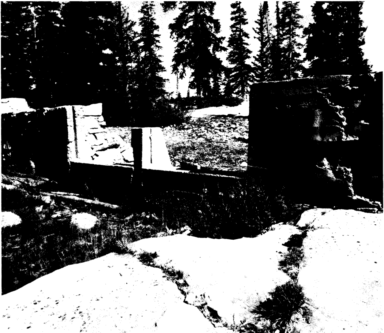
Concrete spillway with freeboards removed at Fire Lake Dam. Poured in-place concrete spillways were commonly constructed for Utah's high mountain reservoirs.
