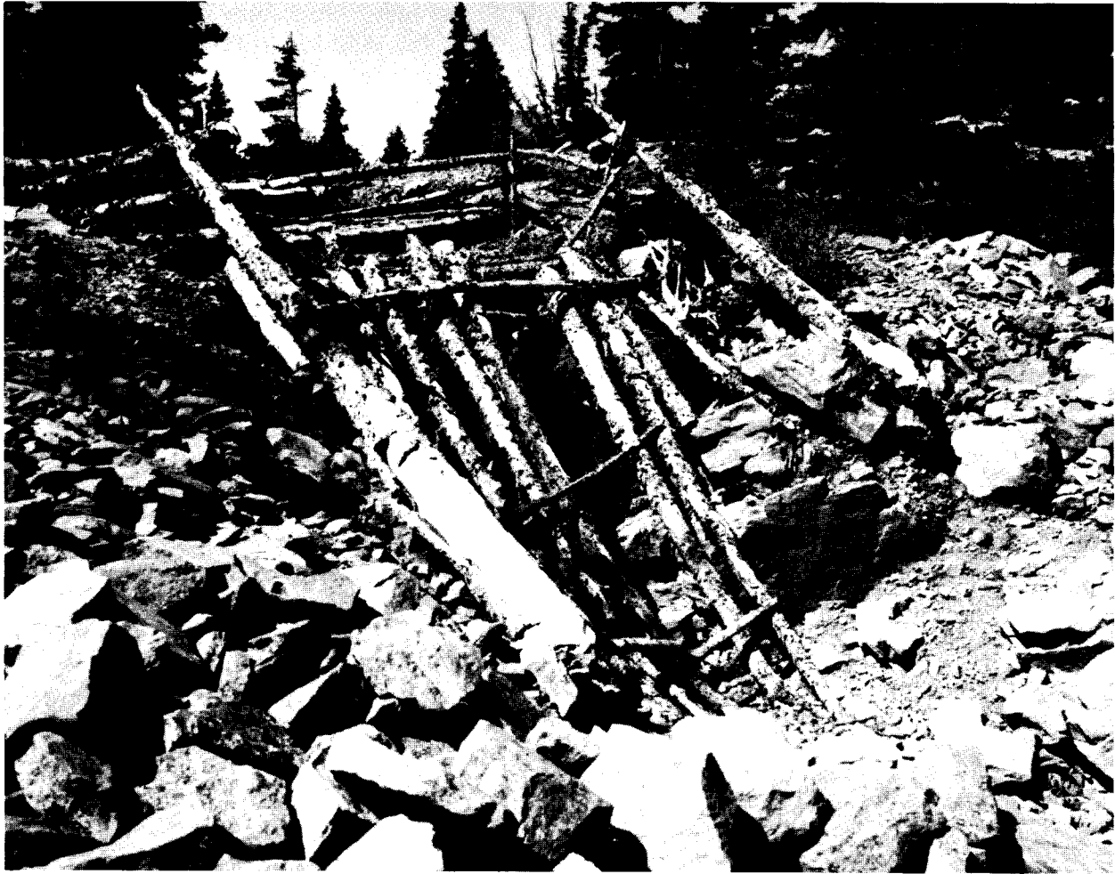
Tunnel intake with log trash rack at Farmers Lake Tunnel. Instead of the typical earth-fill dam, a 300-foot-long tunnel was drifted through the rock of the terminal moraine which lowered the natural lake level by 12.5 feet.
