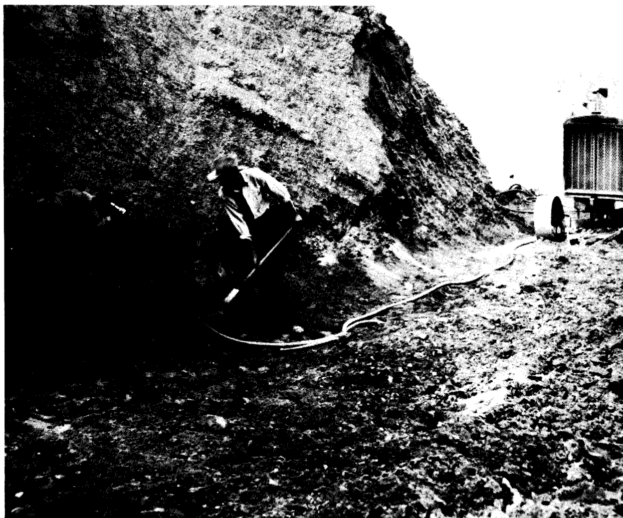
Excavation at Moon Lake Dam. The lake's proximity to an established road allowed workers to utilize more mechanized construction methods such as this pneumatic equipment. (Photograph courtesy of Moon Lake Water Users Association, Roosevelt, Utah, ca. 1934.)
