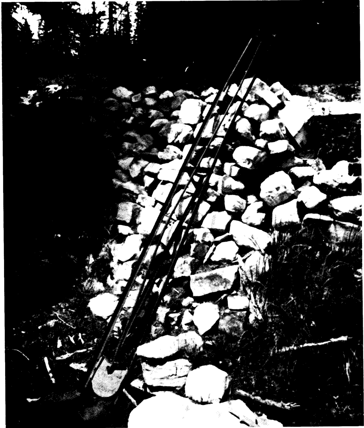
Inclined, shovel-nosed outlet gate, stem, stem guide and wheel, at Pot Lake Dam. Water flow through the outlet was controlled by rotating the gate wheel, which raised or lowered the gate by moving the threaded stem.
