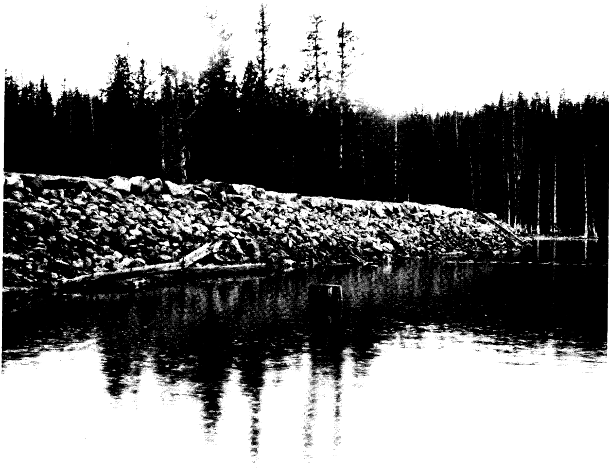
Upstream face of Wall Lake Dam, an obtuse V-shaped structure constructed of a compacted Bentonite clay core, covered with earth and rock fill, and faced with granite stone riprap on both slopes.
