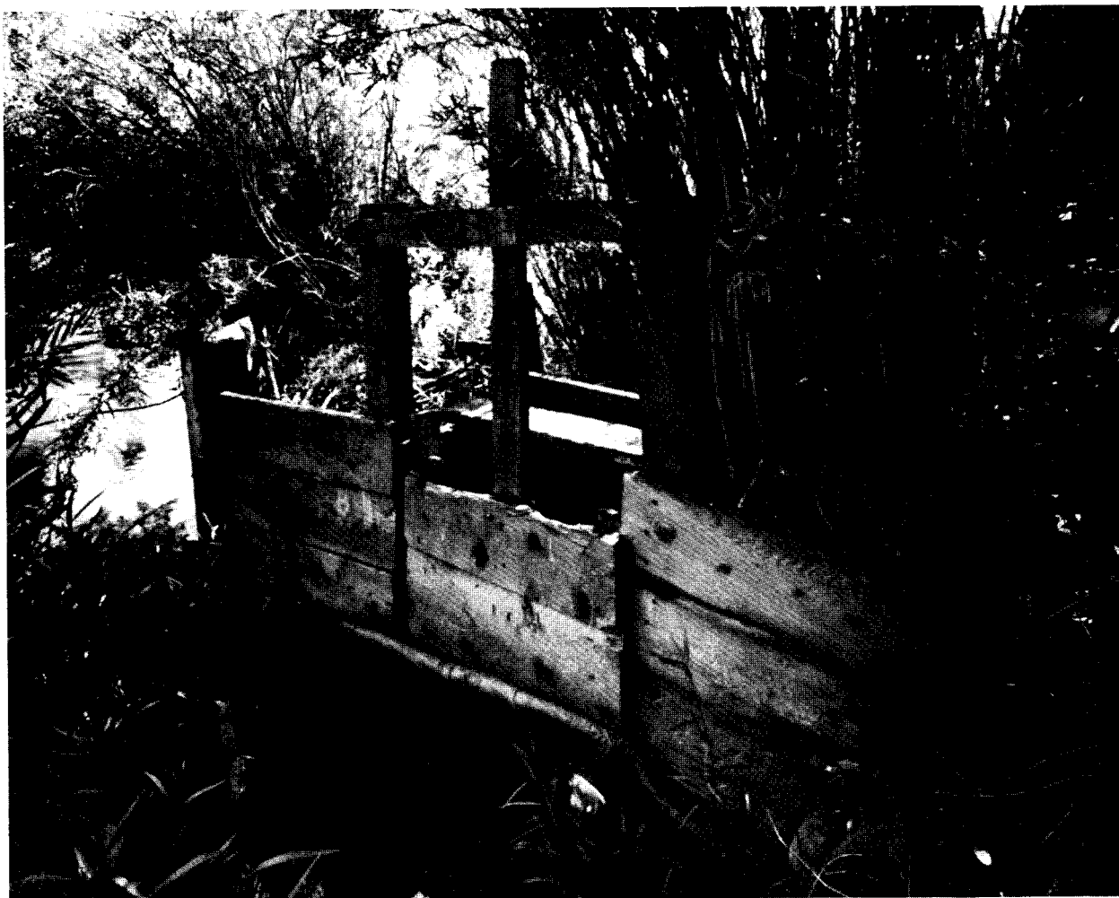
This simple wooden headgate on the Jepp Thomas Canal diverted water from the west bank of the Duchesne River and provided water to Thomas' 128 acre homestead.
