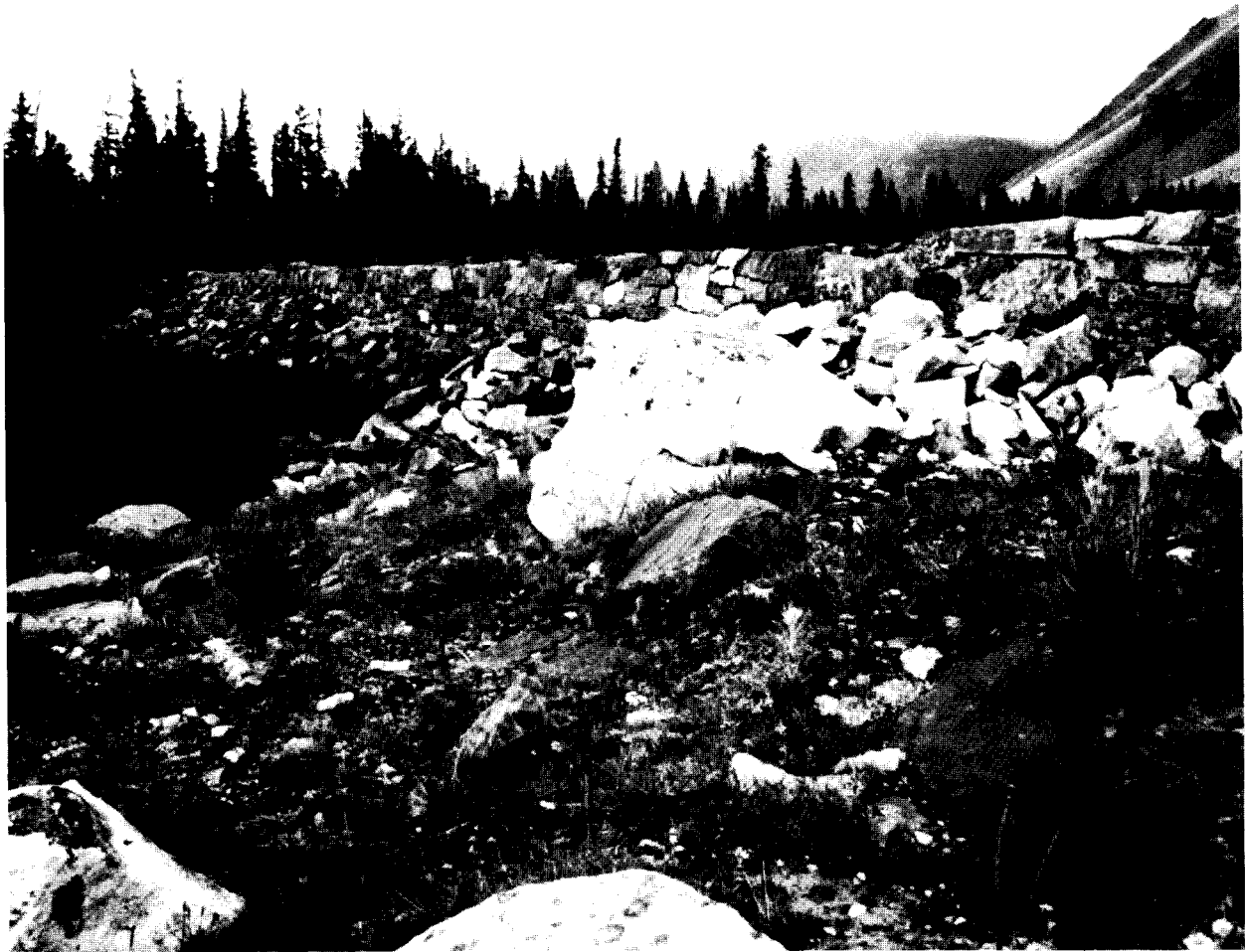
Downstream face of Milk Lake Dam, the only grouted stone masonry dam in the Upalco Unit.
