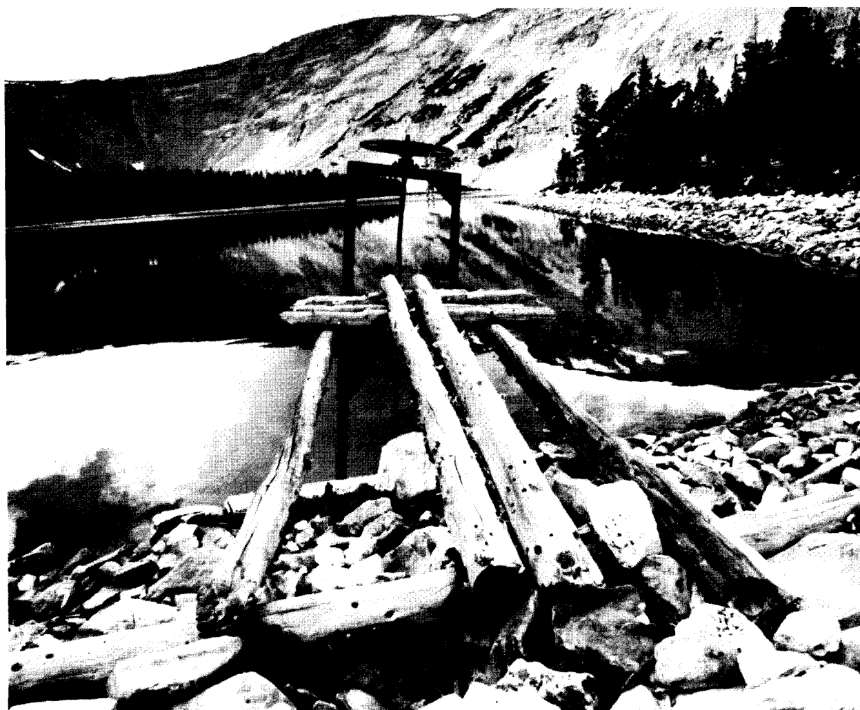
Outlet gate wheel, stem, and stem guide, with log access structure at Bluebell Lake Dam. The dam is representative of small-scale earth-fill construction in the Upalco Unit.
