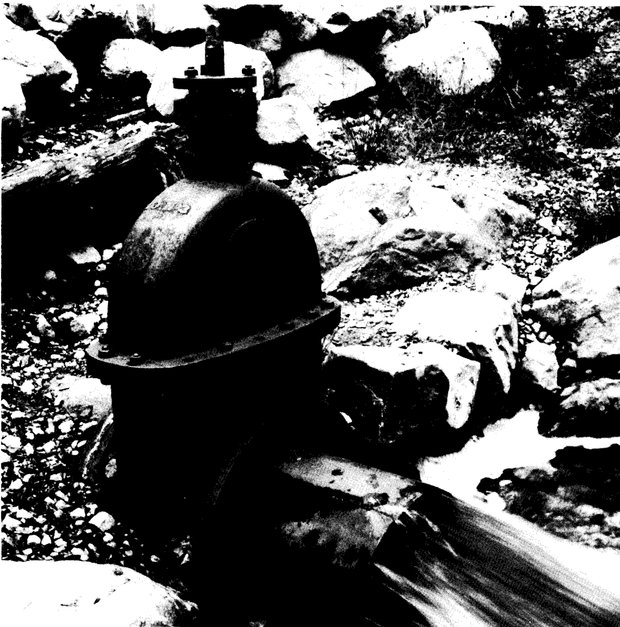
Twenty-inch-diameter Ludlow gate valve, the downstream outlet valve for Trial Lake Dam.
