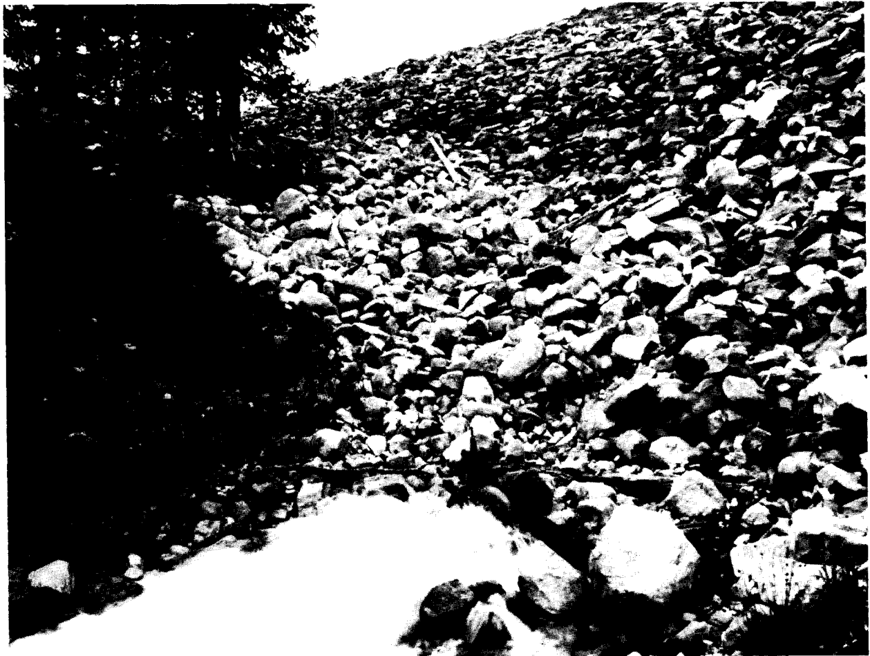
Downstream face and toe of Washington Lake Dam, showing outlet valve. The lake is the largest and most accessible of the fifteen reservoir lakes in the upper Provo drainage. Like Trial Lake, the dam has a concrete core. The unusually steep slope of the walls necessitated hand placement of the riprap stones.
