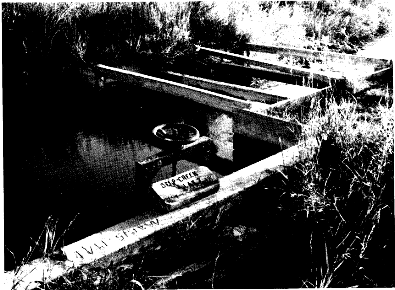
On June 13, 1905, C.G. Hall, Indian Agent at the Uintah Indian Reservation filed for and received the right to appropriate water from the Whiterocks River. When completed, the U.S. Deep Creek Canal stretched for 5,660 feet, was 26- wide on top, and 10-feet wide at the bottom.
